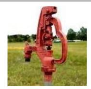
Yard Hydrant – these should have a vacuum breaker or a Reduced Pressure Backflow Preventer to prevent any potential backflow.
