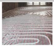
Radiant floor heating – if the system is connected to your home water source, a Double Check Valve Assembly or Reduced Pressure Backflow Preventer is necessary.
