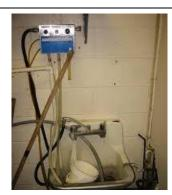
A mop/cleaning sink is present in many homes and businesses. If a vacuum breaker is not installed on the faucet, the non-potable water in the sink could back siphon into the potable water system.
